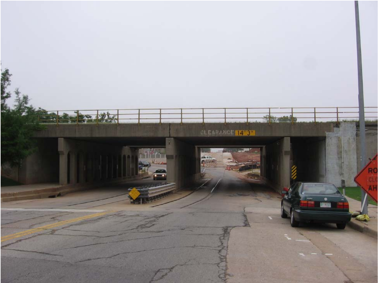
Figure 7. 4 th Street Undercrossing, Looking East
