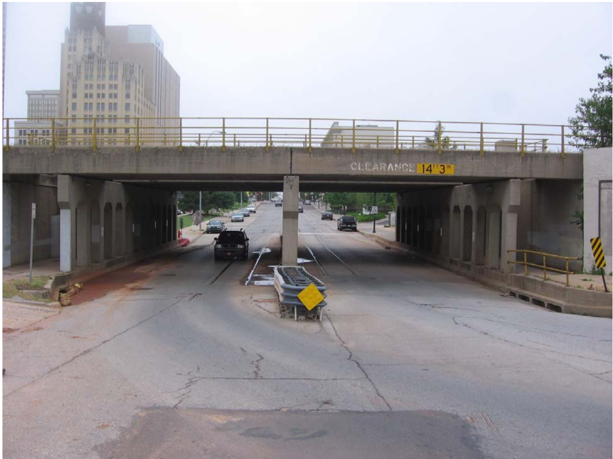
Figure 6. 4 th Street Undercrossing, Looking West
