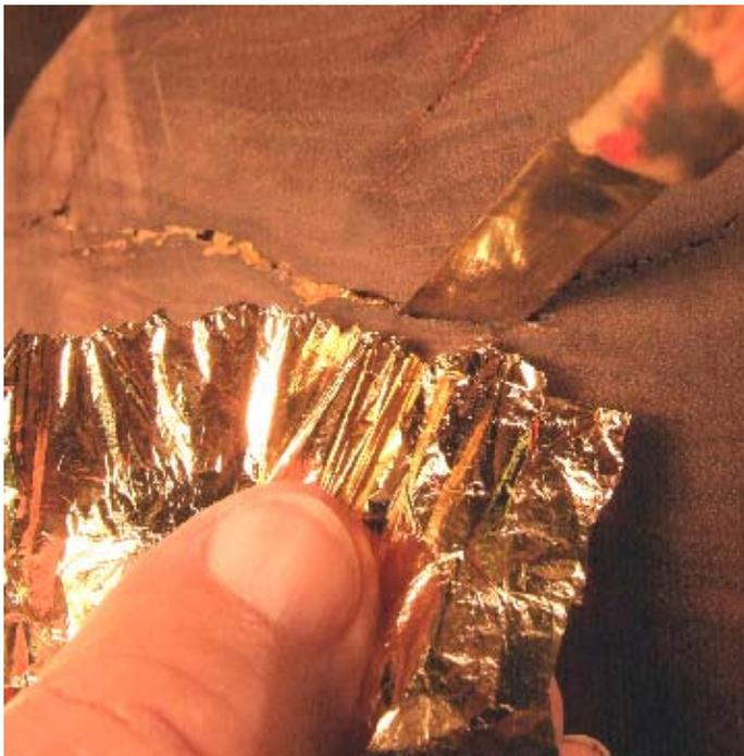
upper right is an inch of brass strip glued into a split in the end of a 1/4" dowel...a sort of mini-spatula. I was amazed at the amount of the very thin foil that could be packed into just a small length of crack! The brown filler at the left is gold mica powder packed in, superglued, and sanded. I figured this would show the contrast with the foil.
