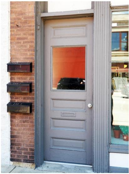
Figure 113: Example of a historic wood stile and rail door with four decorative panels and an upper light in the district.
