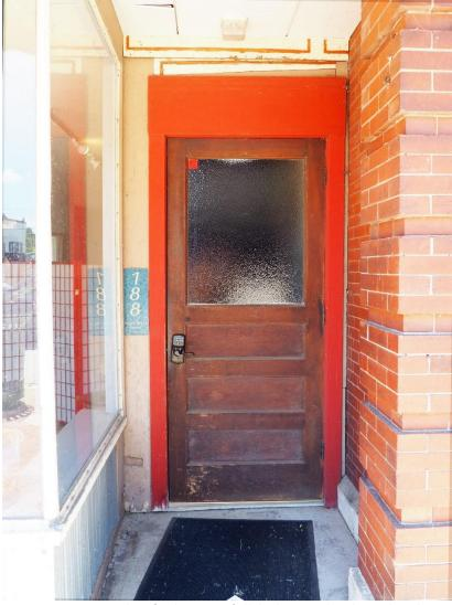
Figure 115: Example of a historic full-light wood stile and rail door with three decorative panels and an upper light composed of frosted glass in the district.
