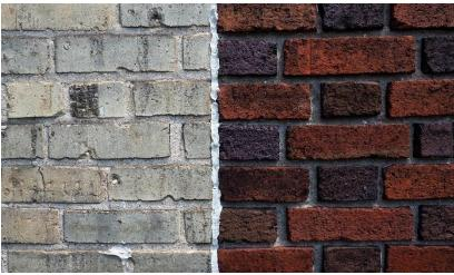
Figure 58: Example of Milwaukee "Silver Fox" common brick at a side façade and a blend of purple dark red, and brown brick at the front façade of a building and in the district.
