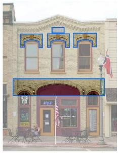
Figure 20: Brick hood molds and inset date plaque.
