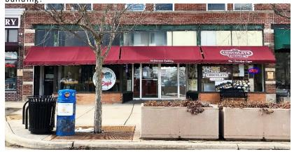
Figure 108: Example of an appropriate contemporary "standard" awning outside of the district that has been inappropriately installed below the masonry opening obscuring and damaging the remaining historic storefront components.
