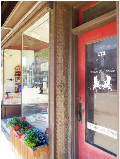
Figure 117: Example of a historic full-light wood stile and rail door and transom in the district with historic tin cladding in the door frame.
