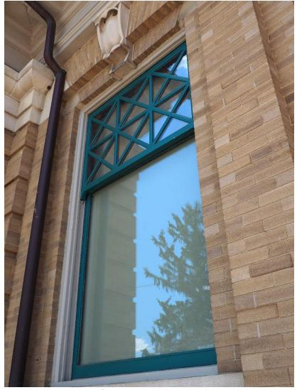
Figure 133: Example of appropriate contemporary wood windows to replicate the original windows which had been previously removed in the district.
