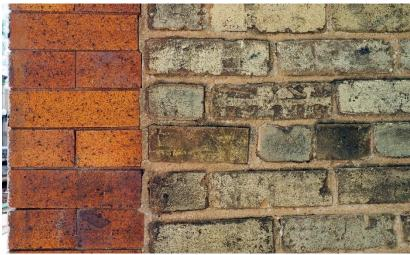
Figure 59: Example of iron spot brick at the front façade and Milwaukee cream common brick at the side façade of a building in the district.
