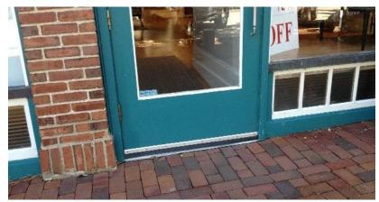
Figure 163: Example of an ADA-compliant threshold not in the district.
