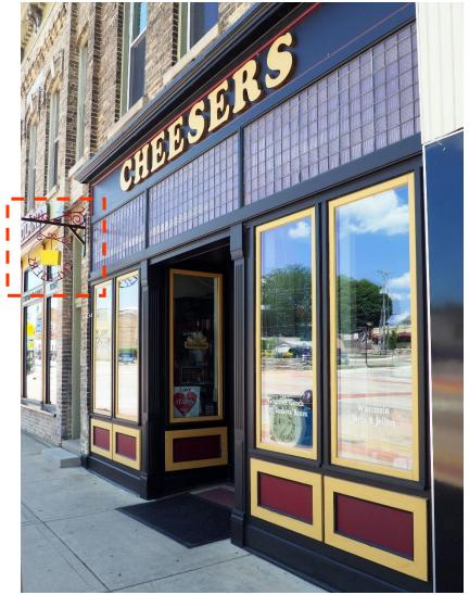
Figure 76: Example of an appropriate contemporary horizontal projecting sign anchored into the masonry mortar joints and individual lettering sign which does not obscure or damage the historic prism glass transoms in the district.
