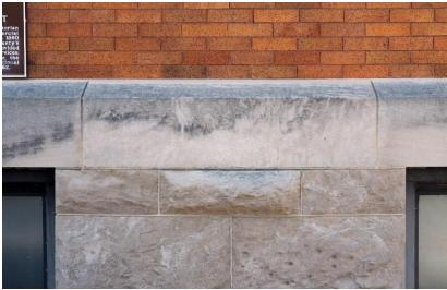
Figure 56: Example of rough-hewn and smooth Indiana limestone at the base of a building with iron spot brick as the exterior wall cladding in the district.
