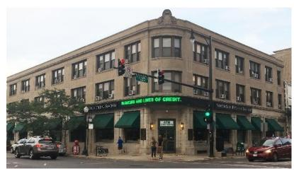
Figure 85: Example of an inappropriate digital banner sign not in the district, that is directly mounted into the building's limestone façade and obscures architectural features at the first floor.
