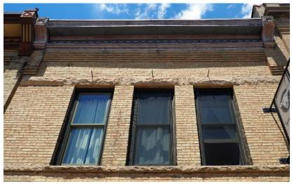
Figure 135: Example of non-historic one-over-one double-hung vinyl-clad wood or vinyl windows in the district.
