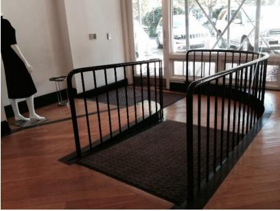
Figure 165: Example of an appropriate contemporary interior ramp in a retail space not in the district.
