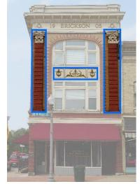
Figure 24: Classical brick pilaster and ornamentation.
