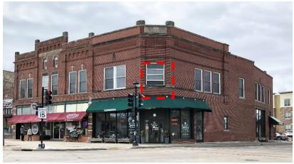
Figure 140: Example of inappropriate contemporary vinyl windows at the second floor and the inappropriate change in the operation style at the center window, not in the district. The original design of the center window is unknown, but based on the date of construction and historic architectural style the four horizontal fixed windows are not appropriate.
