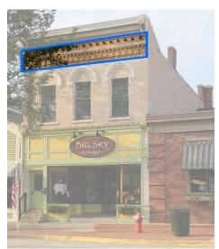
Figure 21: Brick corbeling and relief or pattern work.
