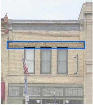
Figure 27: Rough-hewn limestone window headers with bas relief scrollwork carvings.
