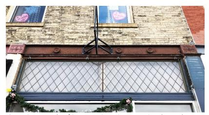
Figure 87: Example of inappropriate sign mounting, located outside of the district, as the sign is directly attached to the historic cast iron header.
