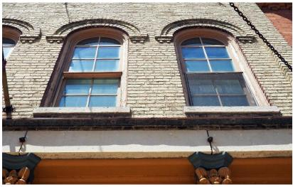
Figure 128: Example of appropriate contemporary wood arched top windows to replicate the original windows which had been previously removed in the district.
