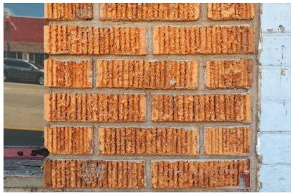
Figure 53: Example of orange brick with a scratched texture in the district.
