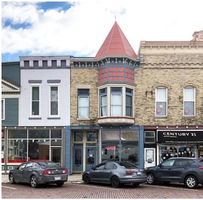
Figure 142: Example of inappropriate contemporary vinyl windows at the second floor, but appropriate preservation of the window opening and operation style, not in the district.
