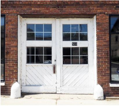
Figure 120: Example of a historic pair of wood stile and rail garage doors with decorative lower panels and upper lights in the district.
