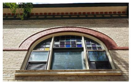
Figure 132: Example of historic tripartite window with a center fixed window flanked by two one-over-one double-hung wood windows with fixed multi-light stained glass transoms.
