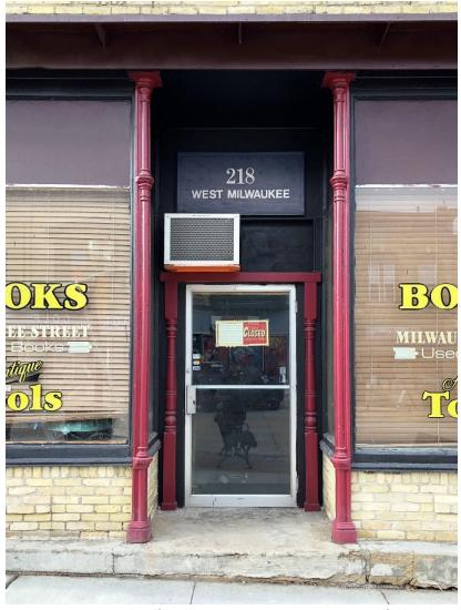
Figure 126: Example of an inappropriate contemporary full-light aluminum door not located in the district. The new door does not fit in the historic opening altering and reconfiguring the historic entrance. Additionally, a historic transom has been replaced with a wood board and a portable air conditioning unit.
