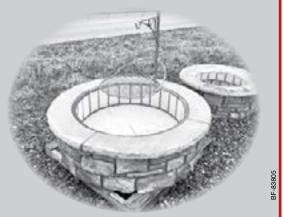
The firepit built for the fire - fully insulated, firebrick lined!
