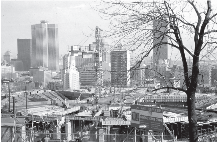
Figure 13.15 | The McIntyre Medical Building under construction, with Place Ville Marie in the left background. (NFOE Inc.)
