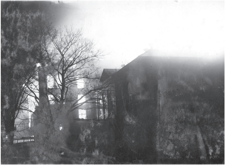
Figure 13.5 | During the fire at the Medical building, McGill University, Montreal, 1907. (MP.1994.15.1.3, McCord Museum, Montreal)
