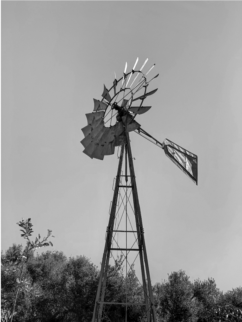
Figure 2.1 Photograph of a Water-Pumping Windmill
