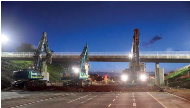
Demolishing Chiltern Gardens footbridge
