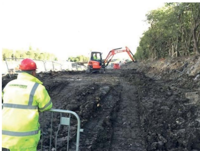
Excavation of embankments between Lobley Hill and Gateshead Quays junction.
