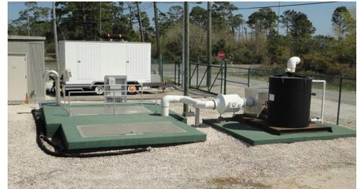
**Zarragossa St. Lift Station (LS #295) Replacement Project** – This project included the replacement of the wet well liner, pumps, the force main connecting the station to the sewer system, and electrical equipment. The entire lift station site was raised for added flood resistance and the project is now complete.
