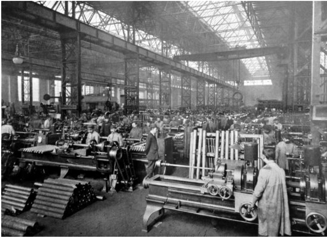
Figure 24.2 Photograph (1899) of AEG large machines factory in Brunnenstrasse (1895–1897), showing a workshop with electrical single motor drive. Oskar Lasche, ‘Die Elektrische Kraftverteilung in den Maschinebauwerkstaetten der Allgemeinen Elektricitäts-Gesellschaft, Berlin’, Z-VDI , no. 5, 43 (1899), 115 (Textblatt 2)
