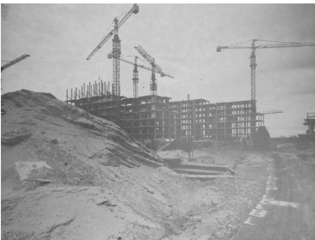
Figure 15.3 One structure during the construction phase of residential Blocks 61–64, New Belgrade. The IMS construction system was made of prefabricated columns and slabs (not panels) and defines the framework and primary structure of the building. Reprinted from: Blokovi 61–64 na Novom Beogradu, prva faza izgradnje [Blocks 61–64 in New Belgrade, the first phase of construction] (Beograd: Gradjevinsko Preduzeće RAD, 1977)
