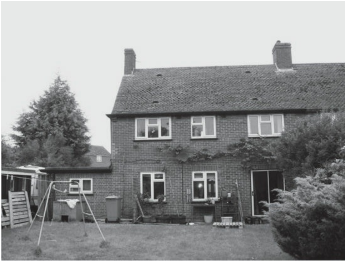
Figure 30.1 Manor Crescent, before refurbishment by ECD Architects. The energy-inefficient house meant that occupants had unaffordable energy bills, were thermally uncomfortable and had health problems. Image copyright ECD Architects. Photograph: Jake Fitzjones
