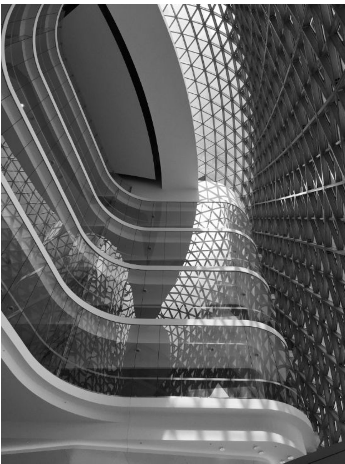
Figure 26.6 Interstitial spaces between successive exterior and interior glazed membranes at SAHMRI. Photograph: Sandra Kaji-O'Grady
