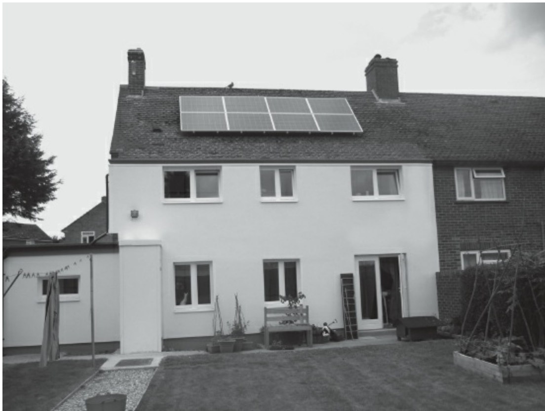
Figure 30.2 Manor Crescent, after retrofit by ECD Architects in 2011, including addition of 220mm externally rendered wall insulation, roof insulation and solar panels on the roof, significantly reducing energy bills (by about 65%) and environmental impact
