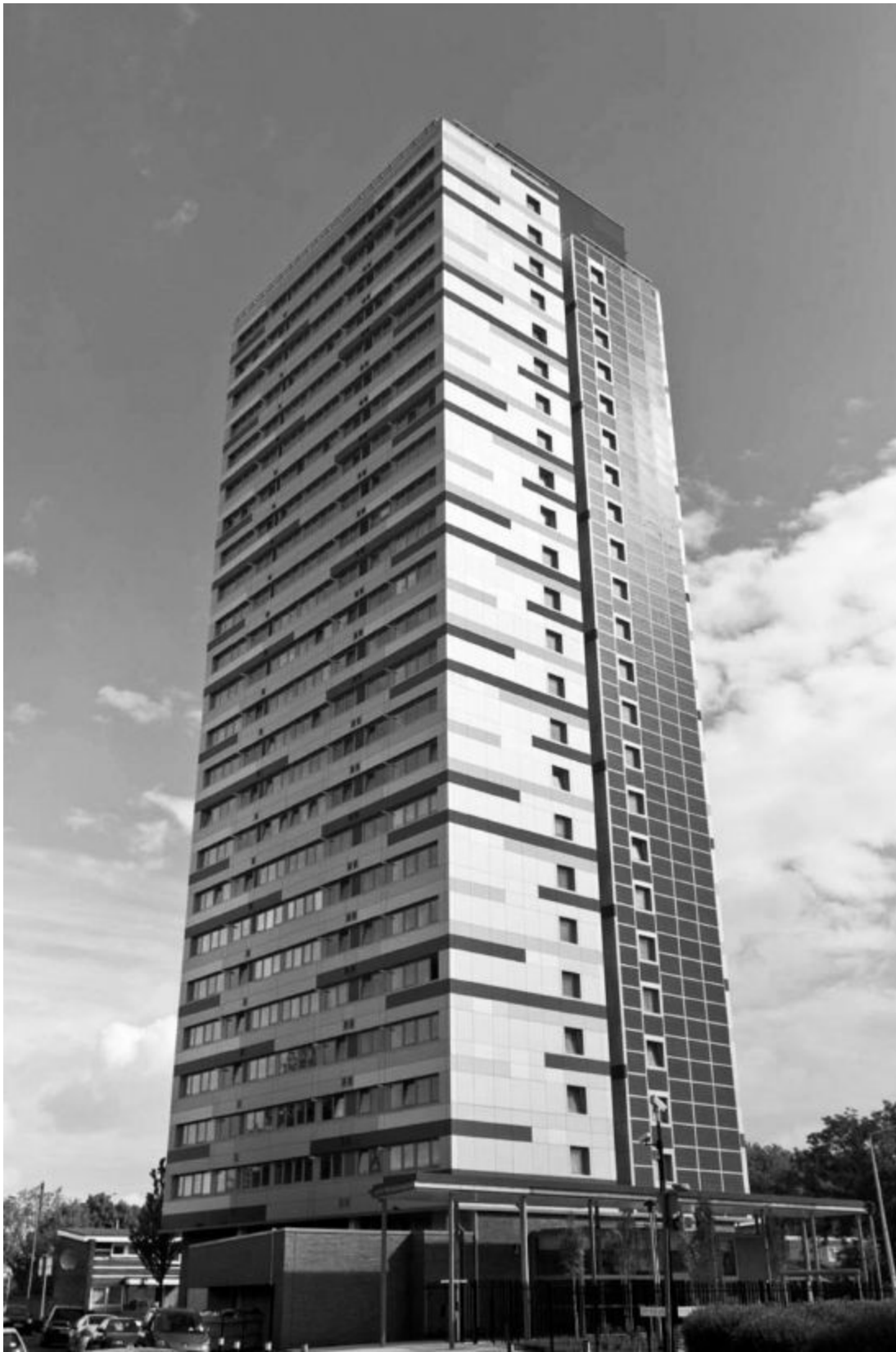
Figure 30.5 Ferrier Point after its energy-efficient upgrade with new windows, externally insulated metal rain screens and 370m 2 vertical PV panels, all installed while residents remained in situ . Image copyright ECD Architects. Photograph: Jake Fitzjones
