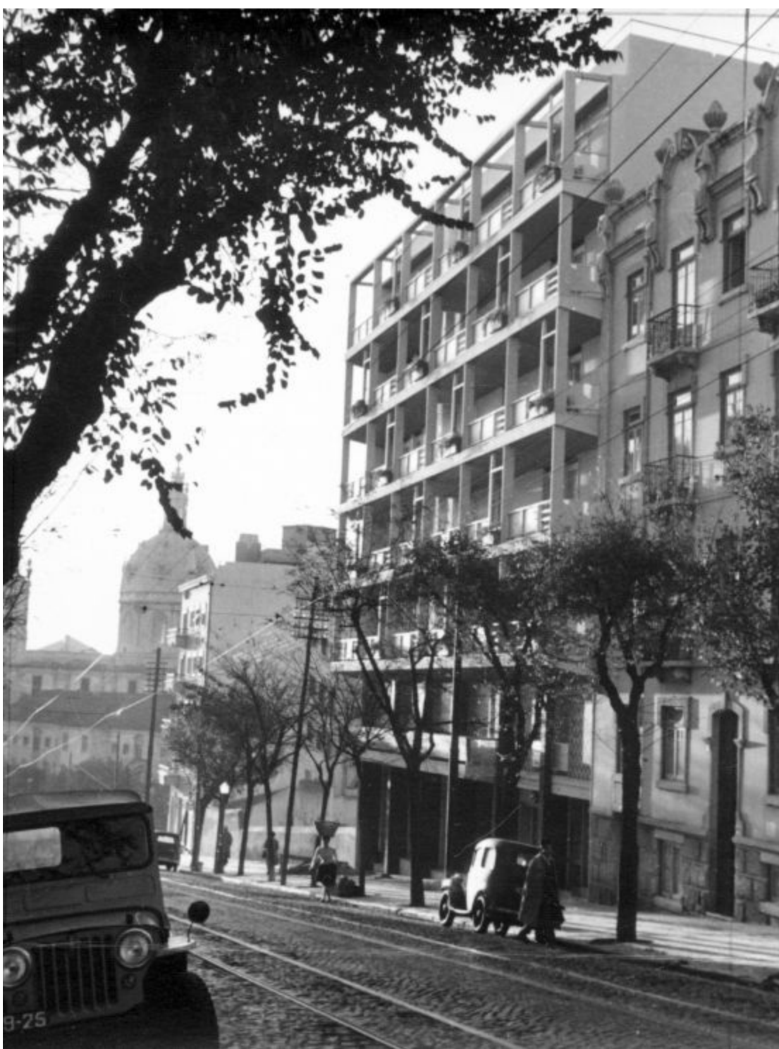
Figure 21.2 Arch. Manuel Laginha, multi-family house in Rua Domingos Sequeira 11, Lisbon (1952–1954). View of the street elevation, with the Estrela basilica in the background. Instituto da Habitação e da Reabilitação Urbana, Lisbon
