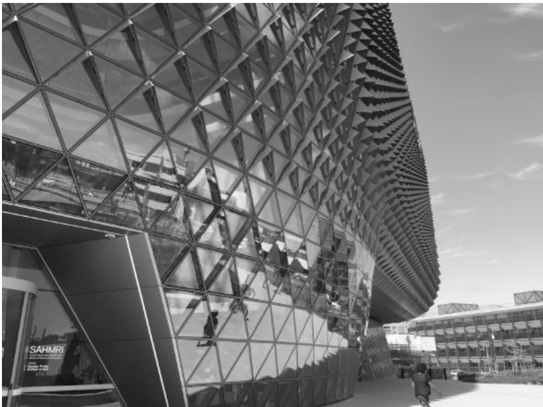
Figure 26.3 SAHMRI exterior. Photograph: Sandra Kaji-O'Grady
