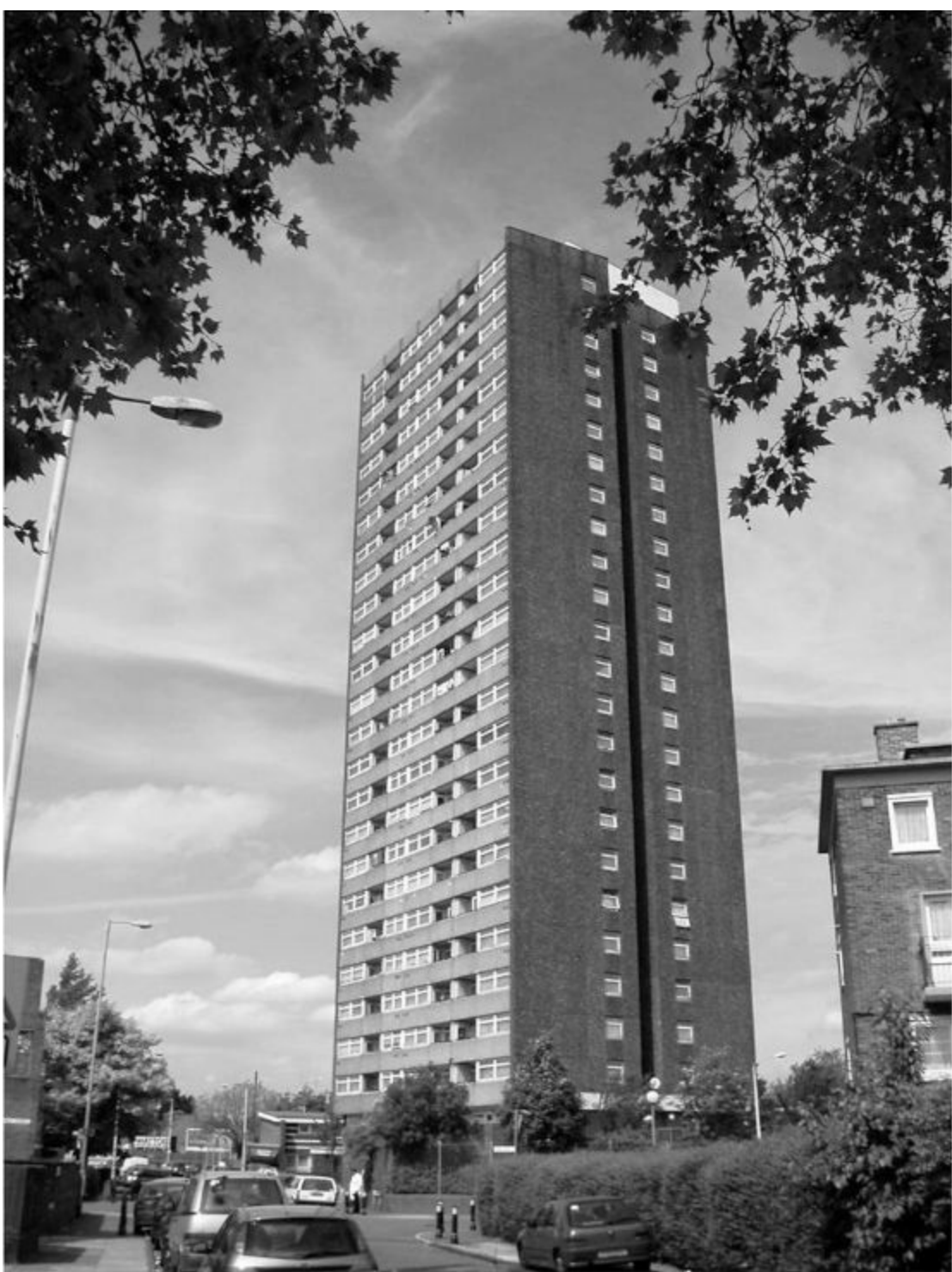
Figure 30.4 Ferrier Point is a 23-storey, 1968-built residential tower in Newham, London, one of the few of its kind to have not been demolished. Can the need for sustainable retrofit also be an opportunity to enhance the architectural quality of the building? Image copyright ECD Architects. Photograph: Jake Fitzjones
