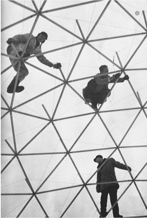
Figure 21 Geodesic dome under construction. Note the pentagon, center-left. Courtesy of The Estate of Buckminster R. Fuller.
